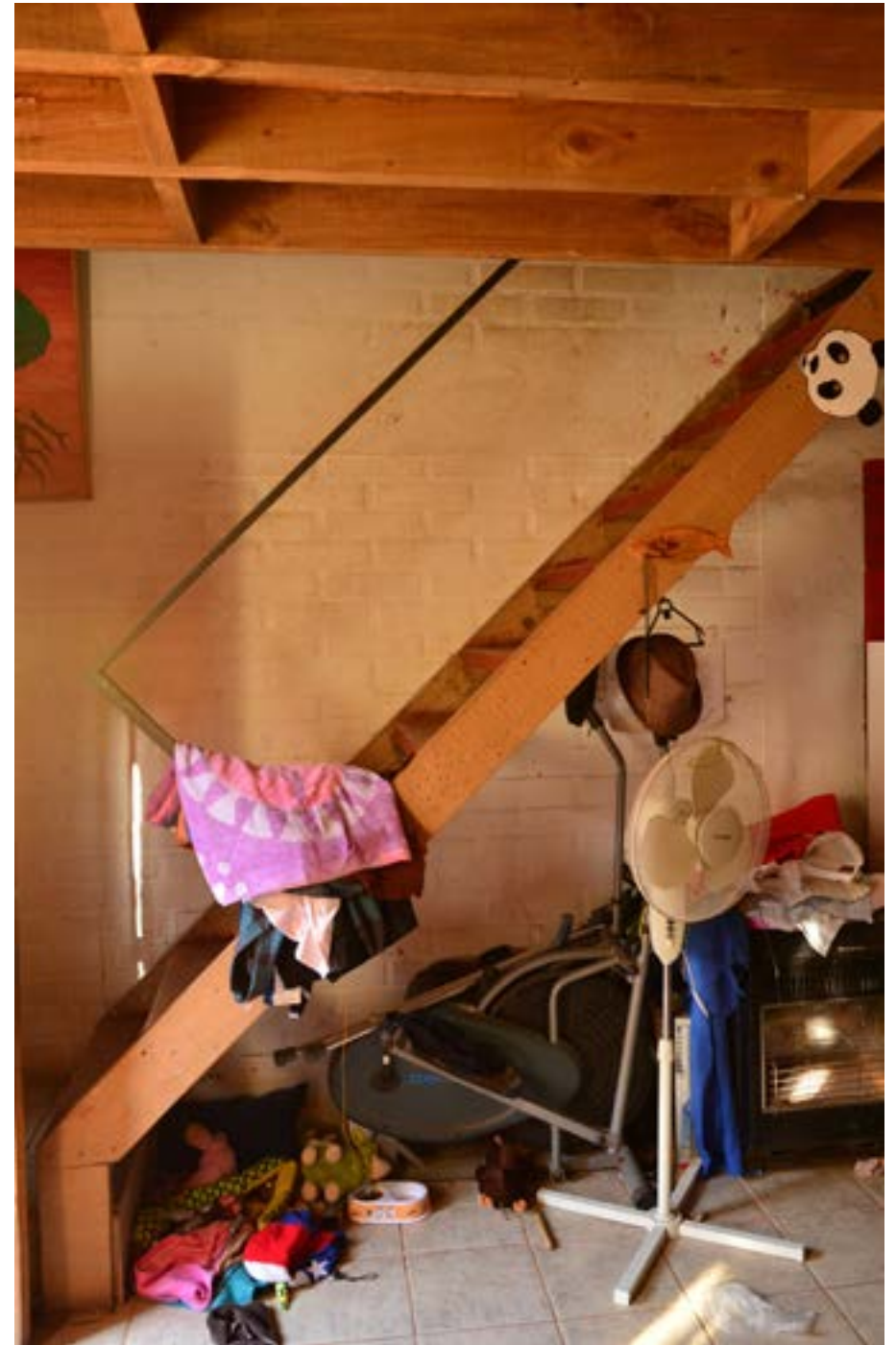
Staircase made with wood
