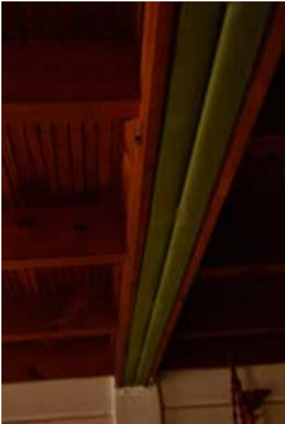
Steel beam for floor additions
