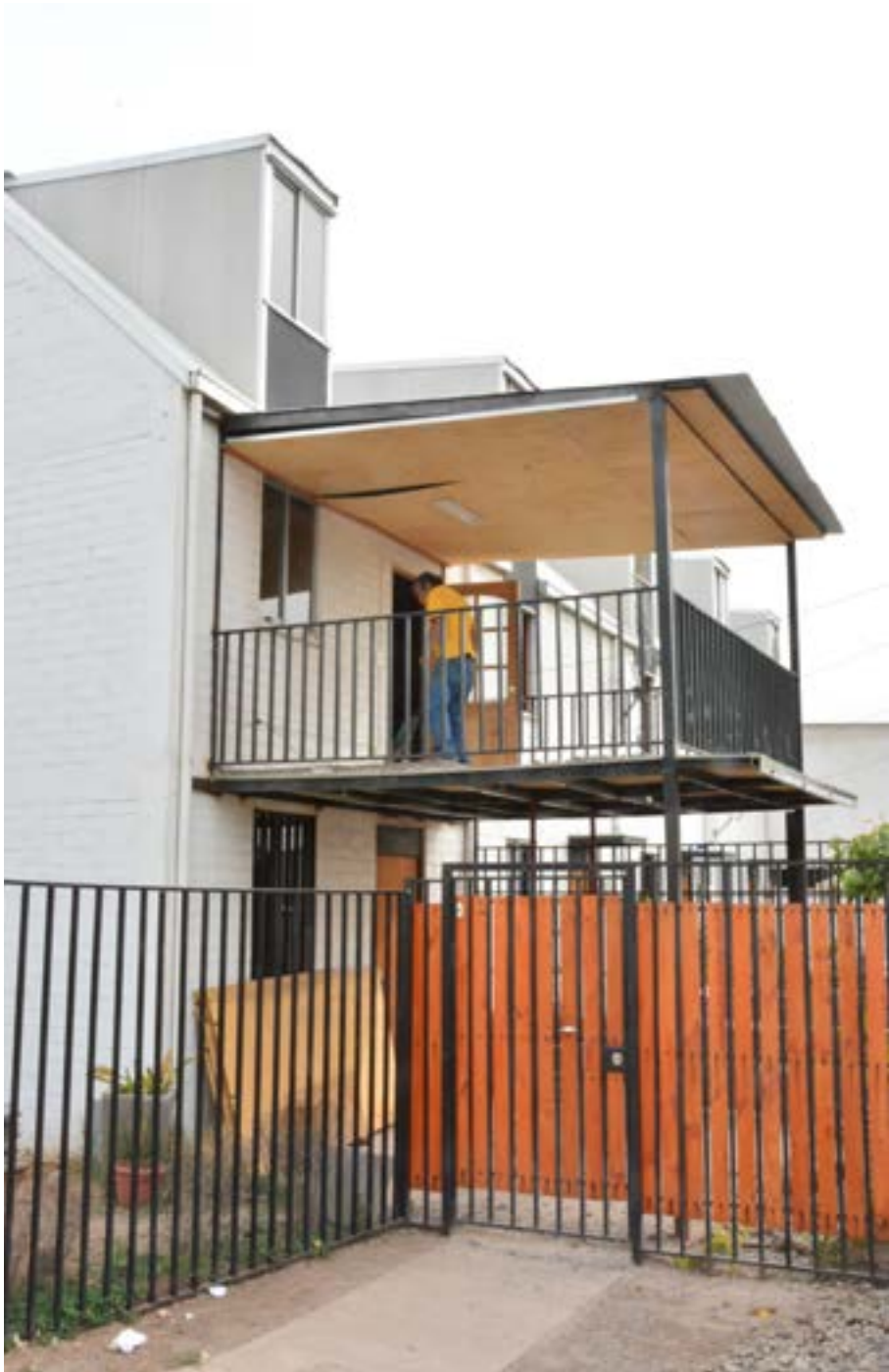
Steel Structure Expansion being demolished
