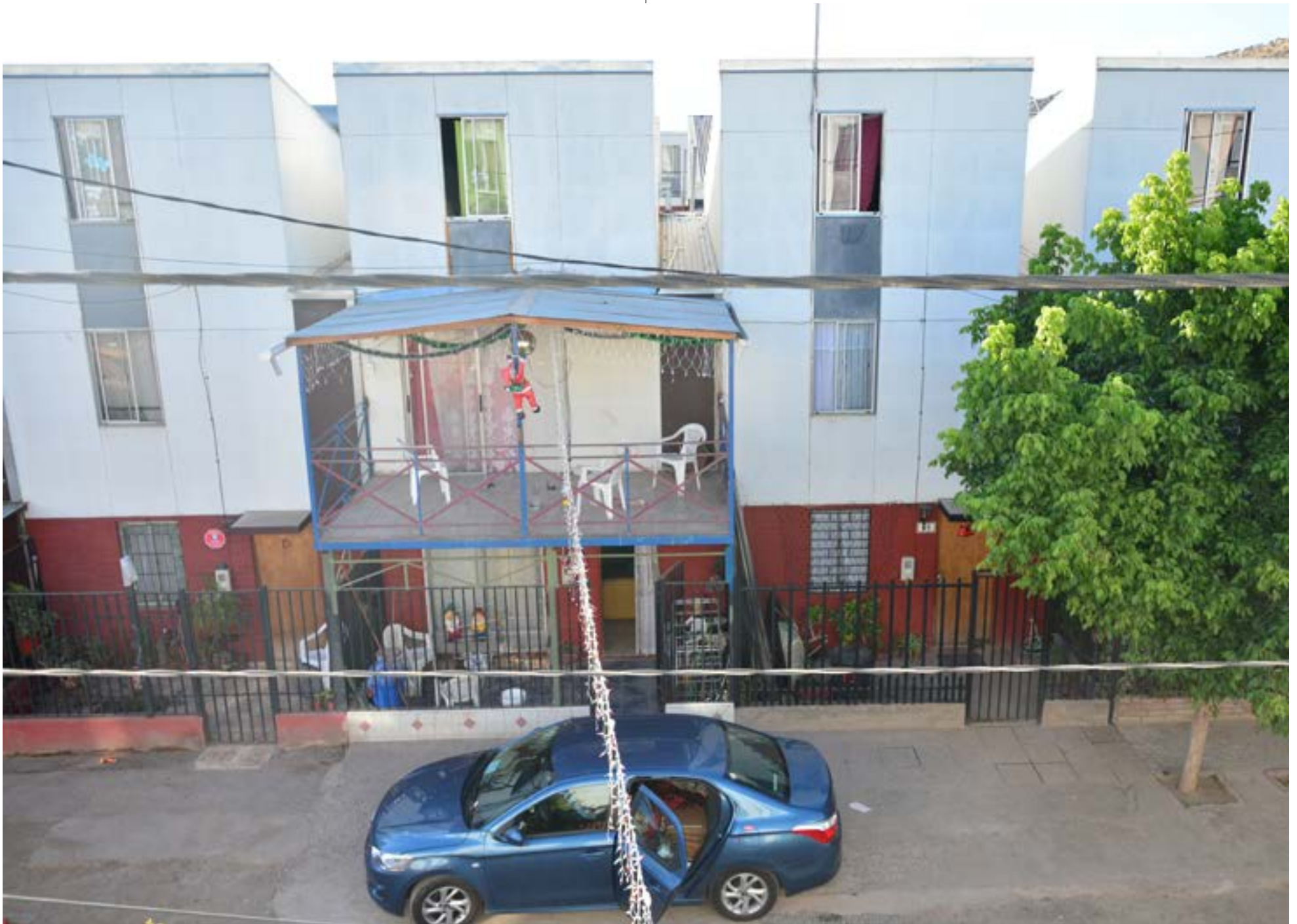
Houses facades with additions
