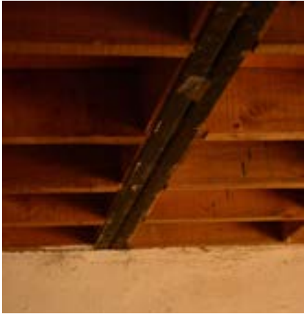
Steel beam and wooden floor
