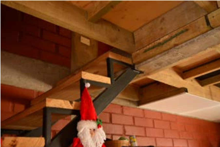
Staircase and Structure
