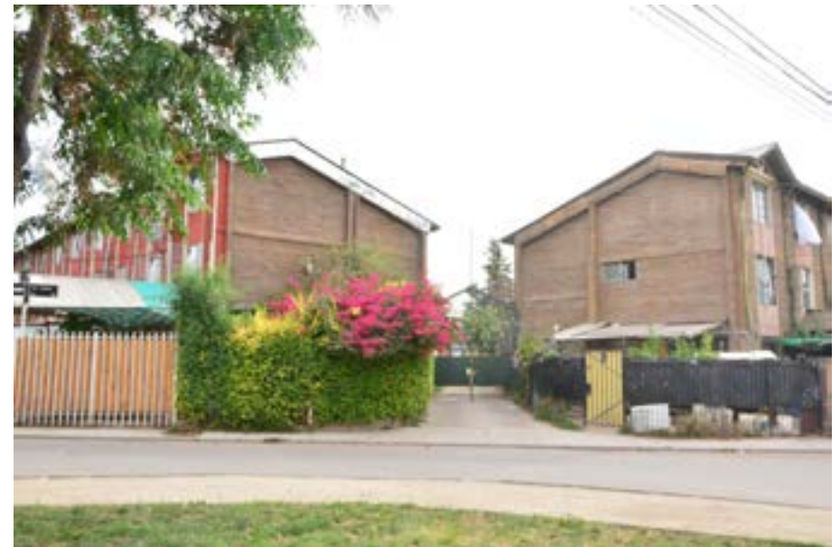
Corner entrance to macro block
