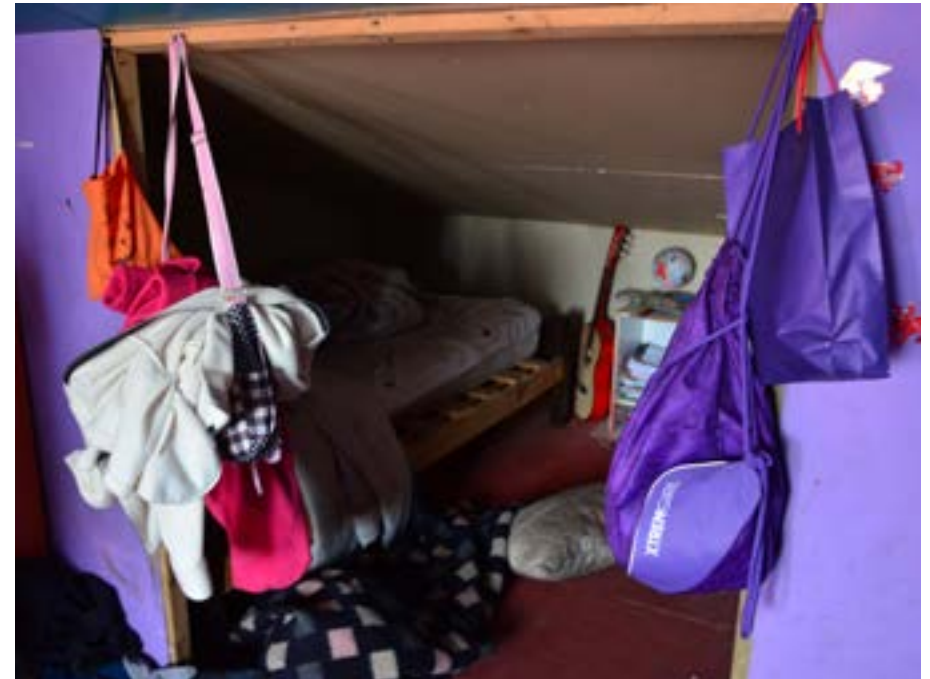
Additional room below tilted roof
